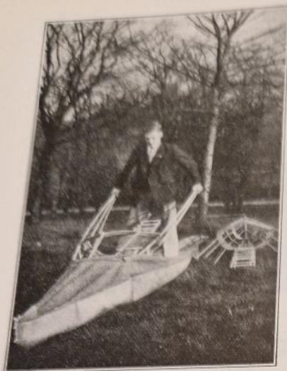
Assembling a Folding Boat.
