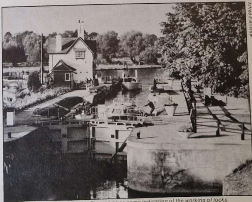
This picture of Goring-on-Thames gives some indication of the working of locks.
